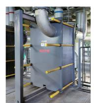
**Heat Recovery** with the Wort Pan **Condenser (Example)**
